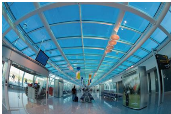
Brazil: TROX swirl diffusers distribute fresh air to the halls and corridors of Rio de Janeiro's Santos Dumont Airport.
